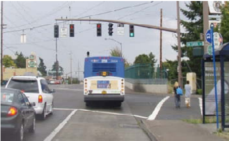
Queue-bypass lane with separate signal phase giving priority to the bus Portland, OR
