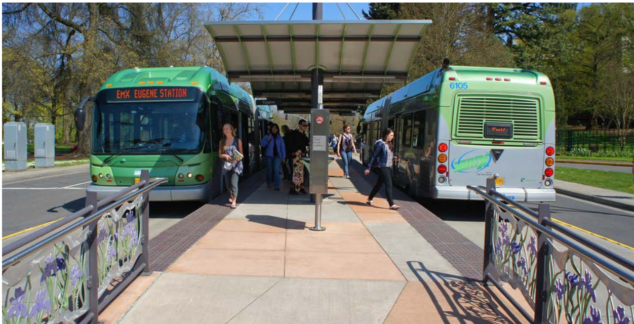
Some elements of EmX include dedicated lanes for buses, covered bus shelters with placemaking features and ticket kiosks. Photo credit: Wolfram Burner (flickr).
