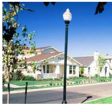
1998 Groundbreaking Single-family and attached housing One and two stories
