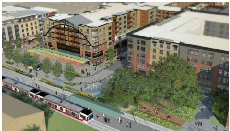
The Orenco Station TOD. Top image: The (relatively low density) main street, built in the late 1990s. Bottom: The high-density “platform district” built adjacent to the light rail line, in 2015/2016.
